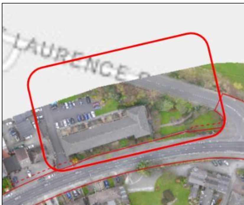
Figure 3-38: Existing aerial view at St. Laurence Glen
