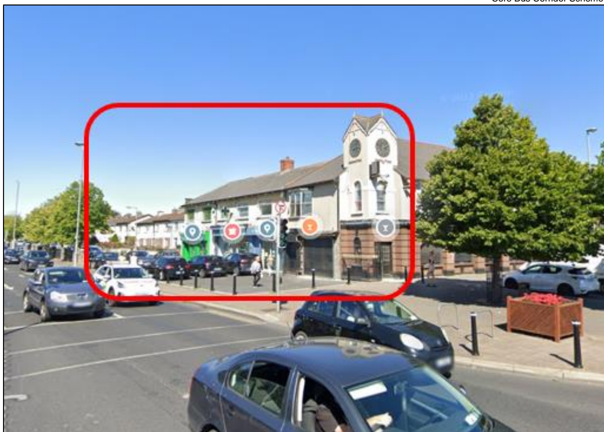
Figure 3-36: Existing Street view at Grange Cross (Image Source: Google)
