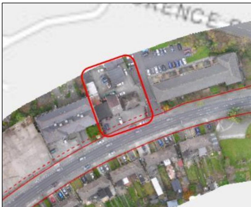
Figure 3-74: Existing aerial view at 5 Ballyfermot Road
