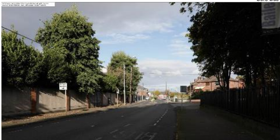
Figure 3-5: Existing conditions at the Steeples, Ballyfermot Road
