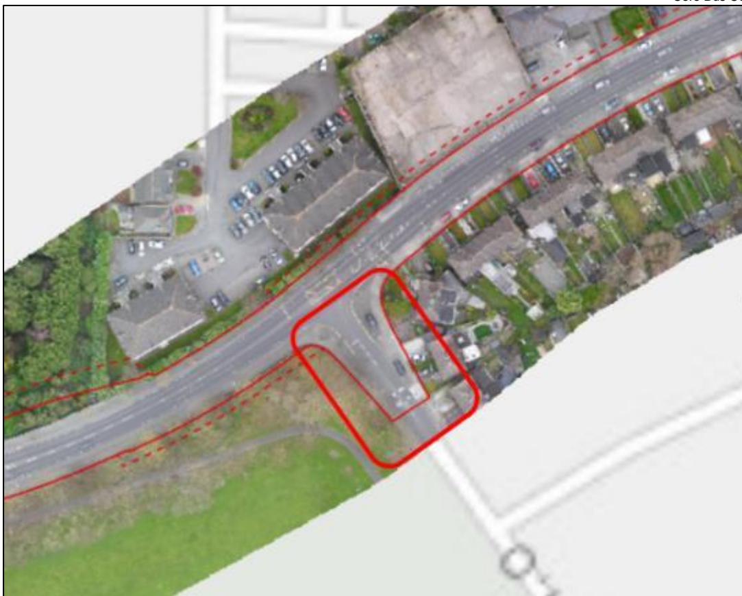
Figure 3-47: Existing aerial view at O'Hogan Road
