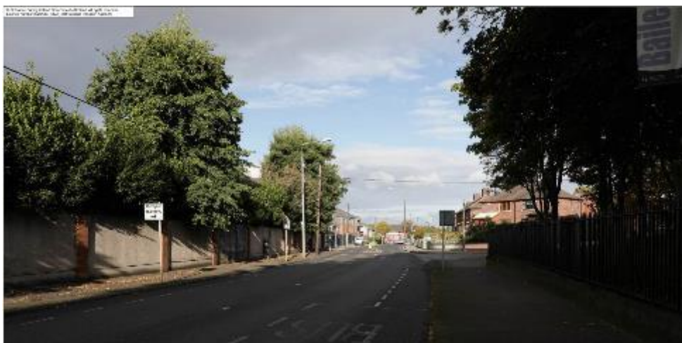
Figure 2-45: Existing conditions at the Steeples, Ballyfermot Road
