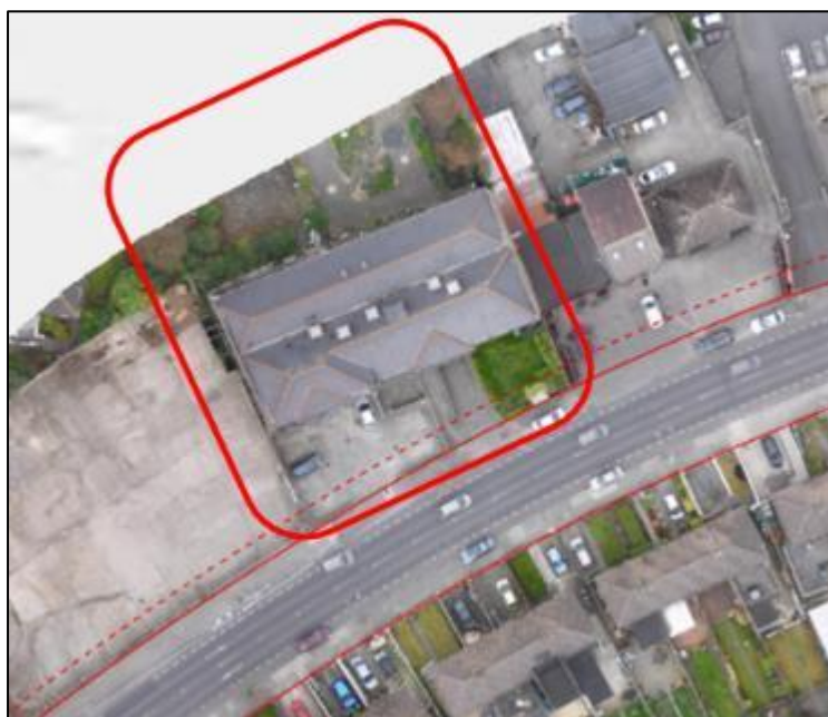
Figure 3-26. Existing aerial view at St. Laurence Court
