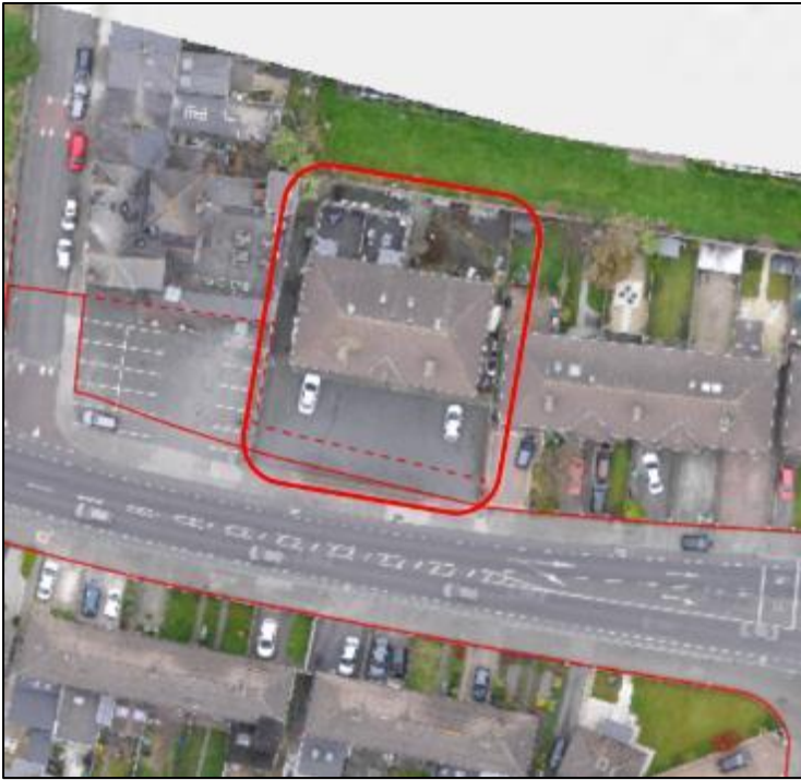
Figure 3-61: Existing aerial view at 3/3A Meadowview
