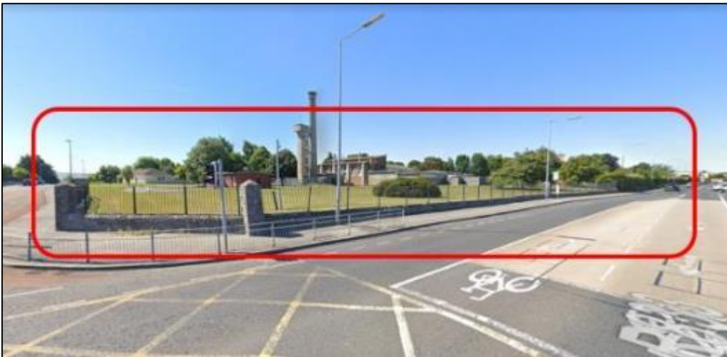
Figure 3-45: Existing Street view of Cherry Orchard Hospital (Image Source: Google)
