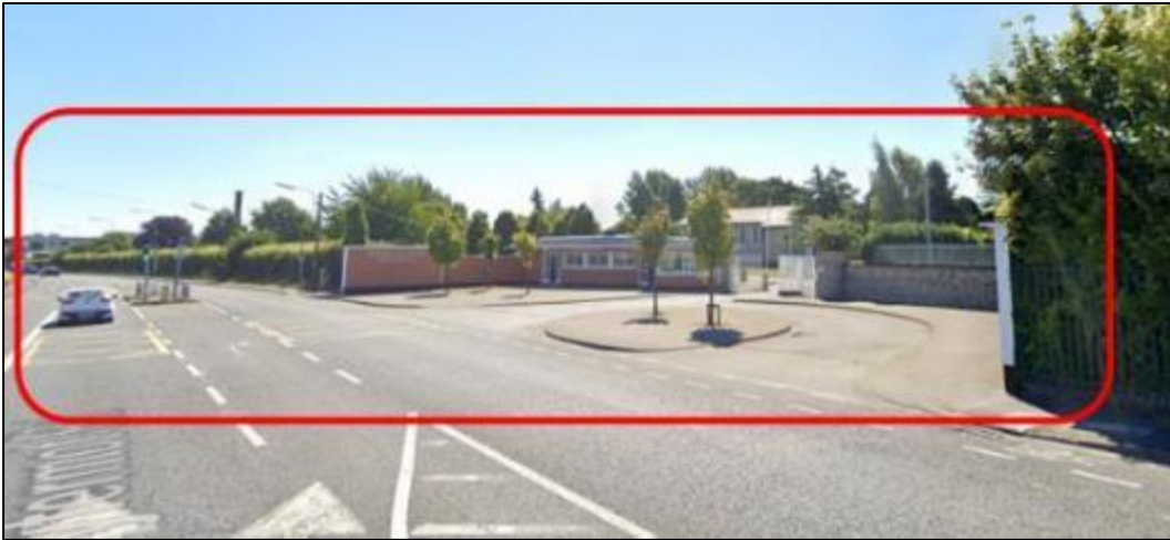
Figure 3-44: Existing Street view of Cherry Orchard Hospital (Image Source: Google)
