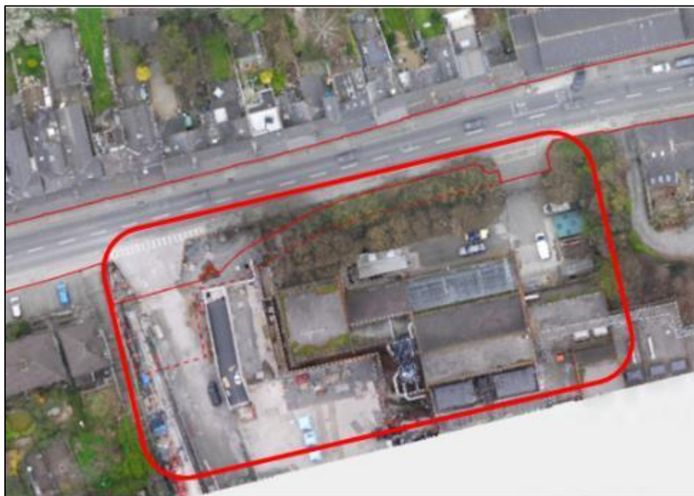
Figure 3-65: Existing aerial view at the National Children's Hospital Access
