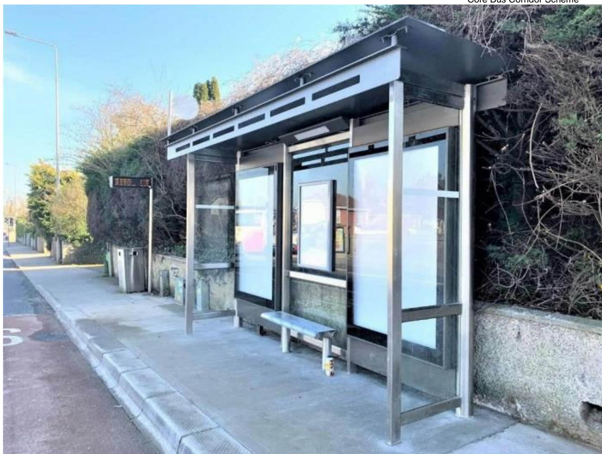
Figure 2.9 Example of a 3-Bay Reliance Cantilever shelter with a narrow roof configuration with and without half end panels.
