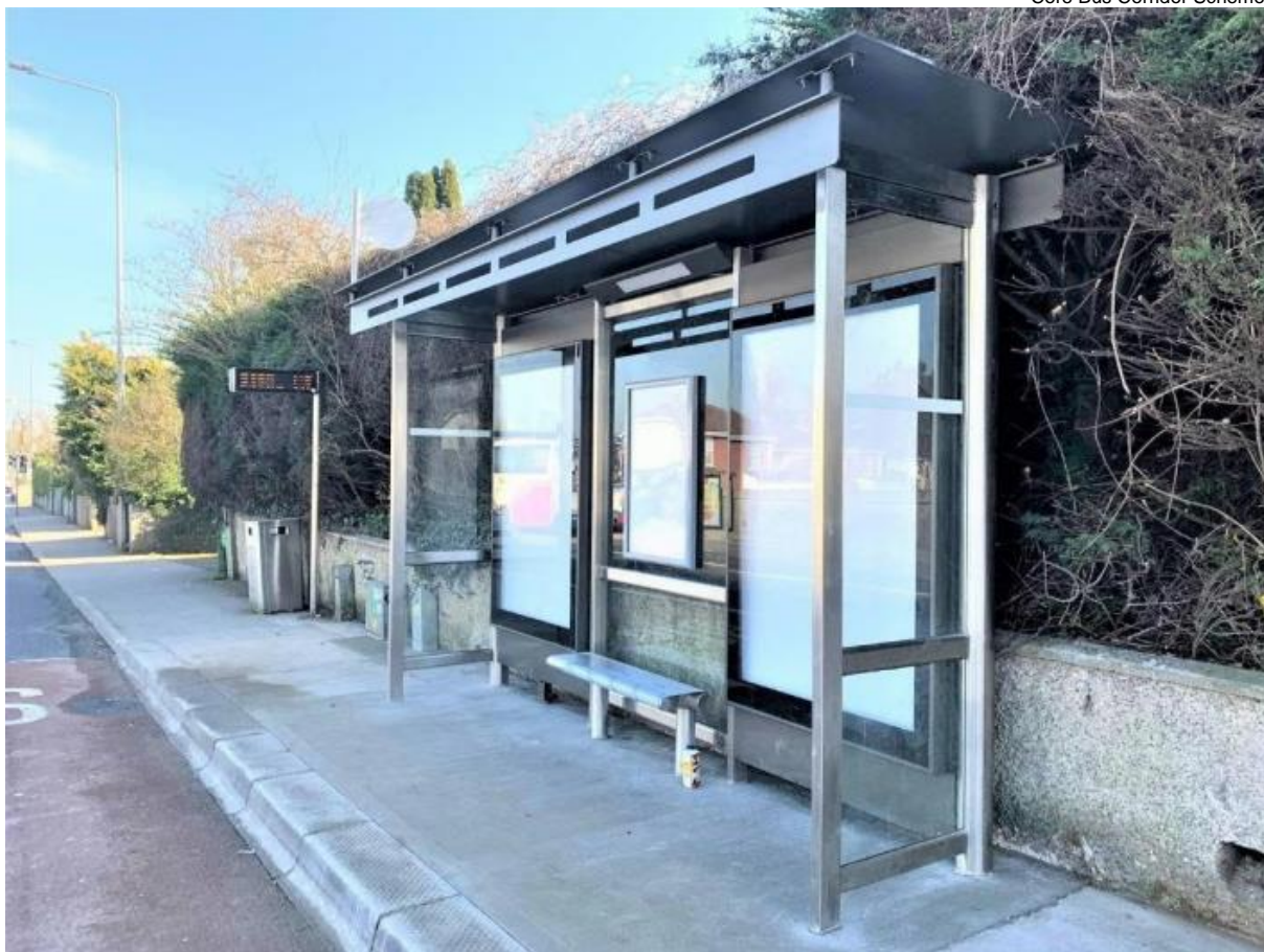
Figure 2.11 Example of a 3-Bay Reliance Cantilever shelter with a narrow roof configuration with and without half end panels.
