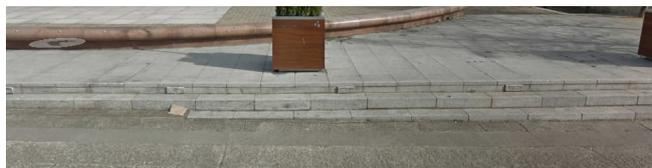
Figure 3.9 Steps - Tripping hazard
